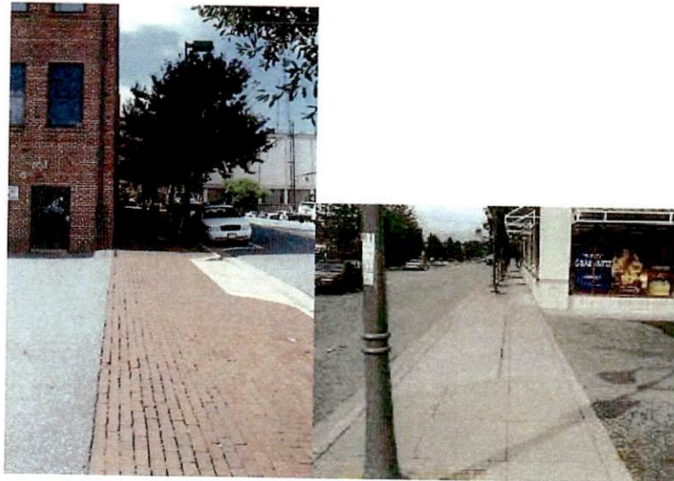
Figure 3-4: Sidewalk Setback from Driveway with Continuous Sidewalk Pattern
