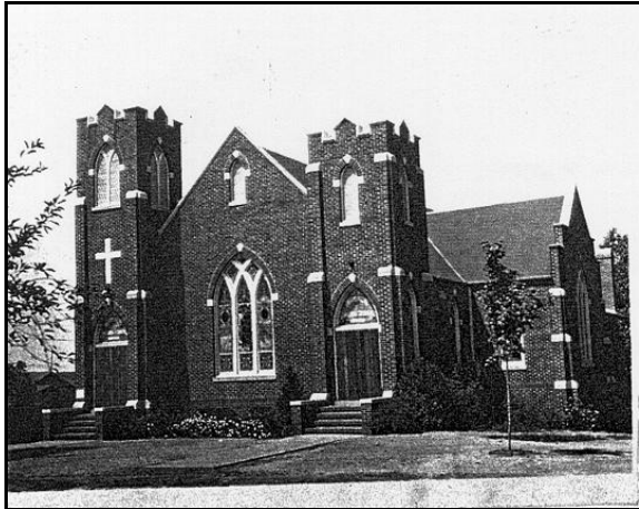
The 1929 Bethany Lutheran Church featured lancet-arched doors and windows, parapeted gables, and a corner tower with a crenellated cornice.
