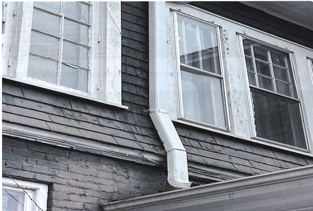
Figure 6: Applicant photo showing current gutters on the house.
